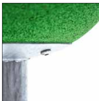
Fixation of Terrasoft floor anchor
